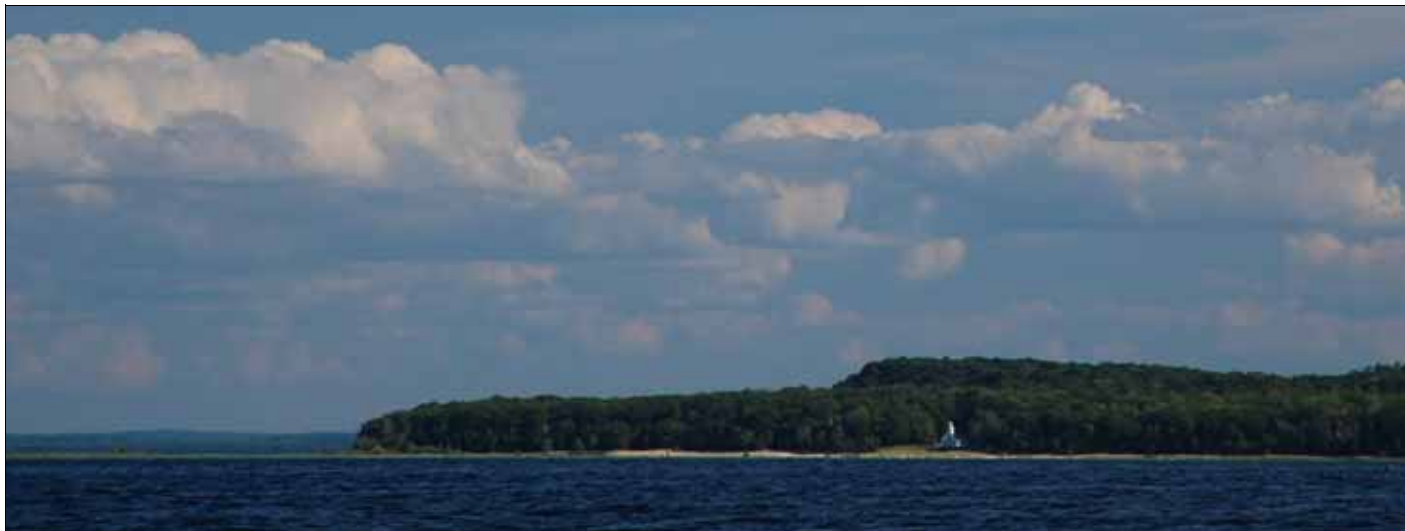
The old Mission Point Light house is surrounded by very shallow water.
